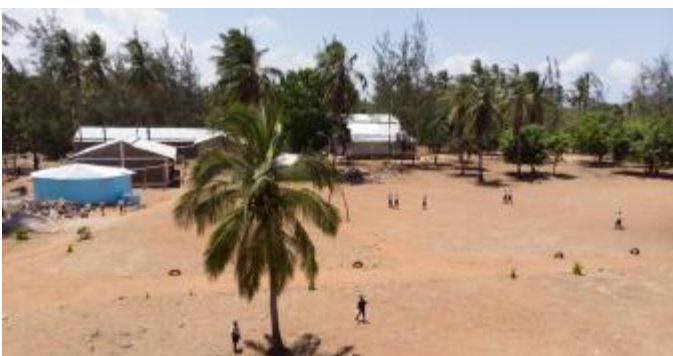
Recently funded water tank at the Chafisi Orphanage
